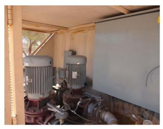
The irrigation booster pump station consists of a VFD, control panel & 2-10HP pumps & motors. The VFD is accounted for separately. The control panel & pumps/motors appear to be original equipment. This component will accumulate funds on a 20 year cycle for the replacement of the control panel & pumps/motors on an "as needed" basis. Once specific pieces of equipment are replaced we can begin accounting for them individually.
