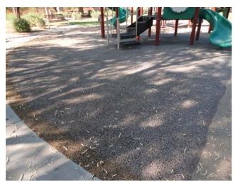
The Tot Turf at this playstructure play area received \$1,336 worth of aromatic urethane coating in 2014, and another coating & repairs in 2017 at a cost of \$2,306.13. This component budgets to replace this Tot Turf in conjunction with the replacement of the playstructure. Accumulated funds should be used for repair work on an "as needed" basis.
