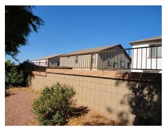
The block walls (148,140 sq. ft.), wrought iron fencing (14,525 sq. ft.) & culvert railings (steel split rail fencing) throughout the community (Parcels 1, 2, 3, 4 & 9) were repainted in mid-2013 by Titan Painting at a cost of \$55,085. This component budgets to repaint these components every eight (8) years. Should the client wish to paint the wrought iron fencing and/or culvert railings on a more frequent basis, we will budget to do so at their request.
