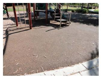
The Tot Turf at this playstructure play area received \$1,173 worth of aromatic urethane coating in 2014, and then was retopped in November 2017 at a cost of \$6,874. This component budgets to replace this Tot Turf in conjunction with the replacement of the playstructure. Accumulated funds should be used for repair work on an "as needed" basis.
