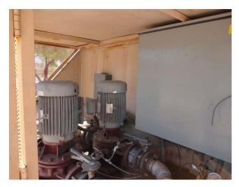
The VFD for the irrigation booster pump station was replaced in October 2013 at a cost of \$3,209.01, and again in April 2018 at a cost of \$3,580.07. This component budgets to replace the VFD on a five (5) year cycle.
