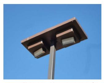
This component budgets to replace the 72-LED light bricks (2) associated with the SolarKing Sentinel lighting system.
