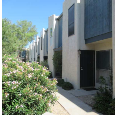
Paint after replacing T-111 siding.
